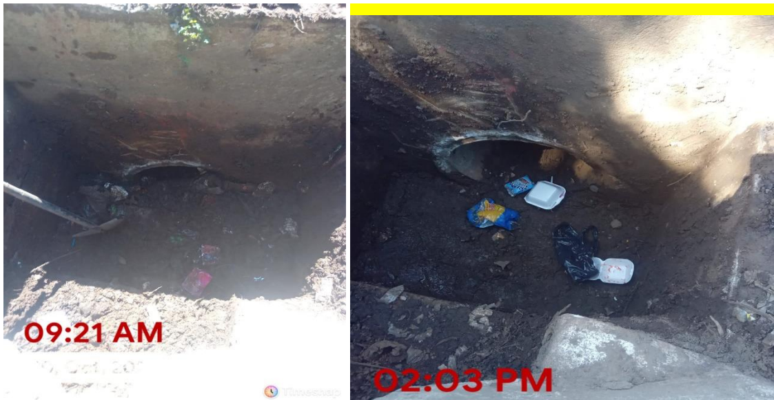
Figure 20: Clearing of storm water drains
